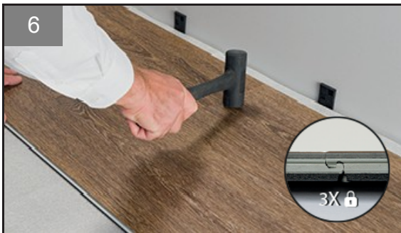
Figure 6: Using a rubber mallet, lightly tap the joint on the short side to engage the locking system.
