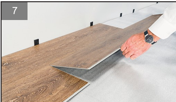
Figure 7: Continue alternating planks on rows 1 and 2. Ensure planks are properly aligned along the chalk line and against the spacers. Finish rows 1 and 2 in this manner, cutting planks at the end of the row as necessary. Ensure that the end planks are a minimum of 6" in length. If necessary, adjust the length of starter pieces to insure minimum plank lengths for each row, with proper end joint stagger row to row.
